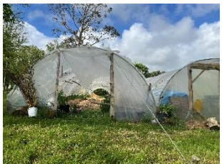
④ Serres tunnel
